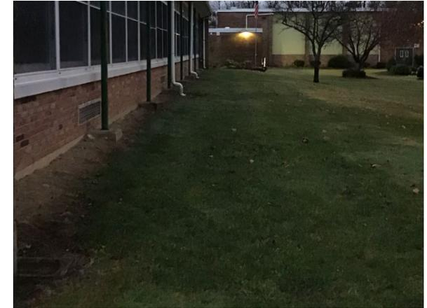
Rain gardens can be installed in the turfgrass areas at several locations around the building by redirecting downspouts into them to capture, treat, and infiltrate stormwater runoff from the roof. A preliminary soil assessment suggests that more soil testing would be required before determining the soil's suitability for green infrastructure.
